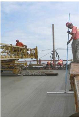
Trapped water/air and elongation of air voids typically occur when finishers apply a finish to the slab before all the bleed water can reach the surface. It can also occur when the ambient conditions of temperature, wind, and humidity result in a high evaporation rate for the bleed water, which causes premature drying and stiffening of the near-surface layer and traps bleed water and air below the surface.
